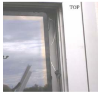
DO Install Glass with Tube in Upper Corner & Pointing Down
